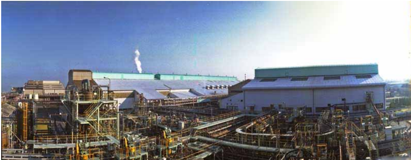
Nickel refinery (Niihama, Ehime Prefecture)
