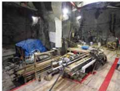
Boring to extract hot water
