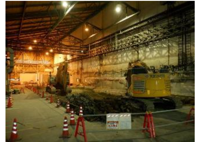
Plant under construction
