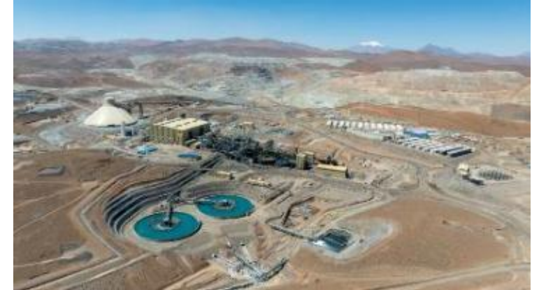
Panoramic view of the Quebrada Blanca copper mine plant
