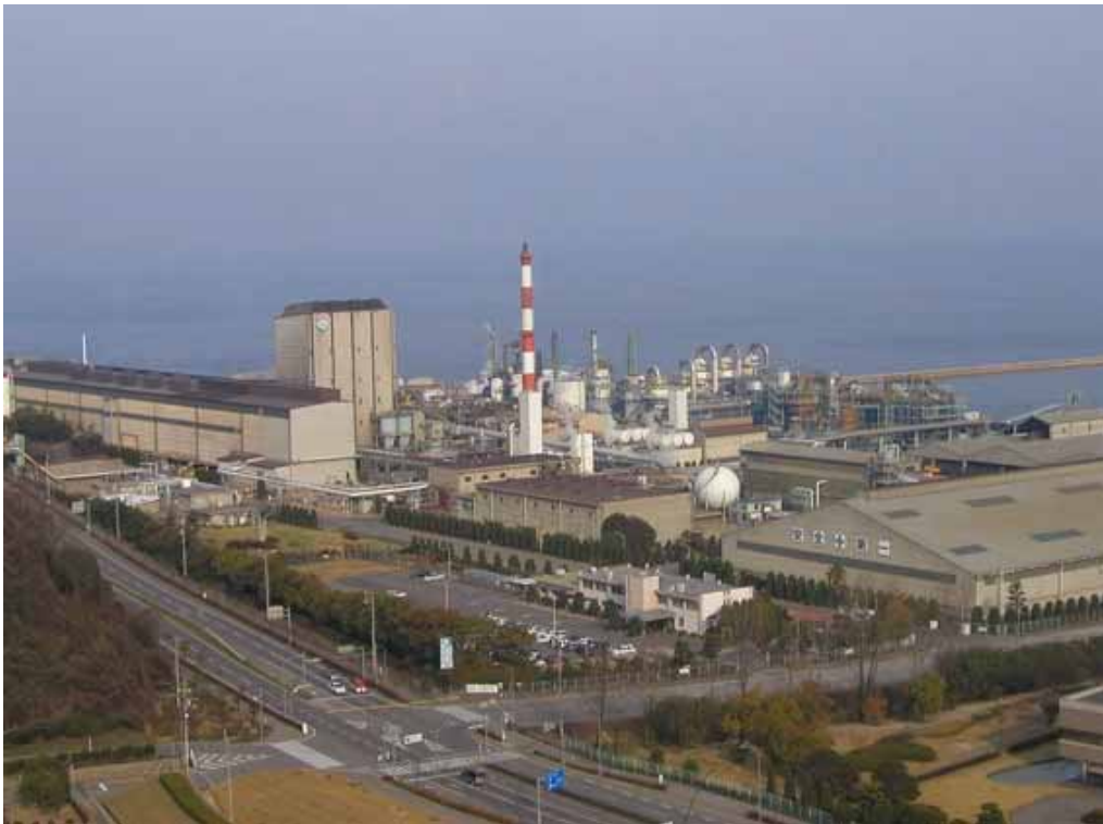
Toyo Smelter & Refinery
