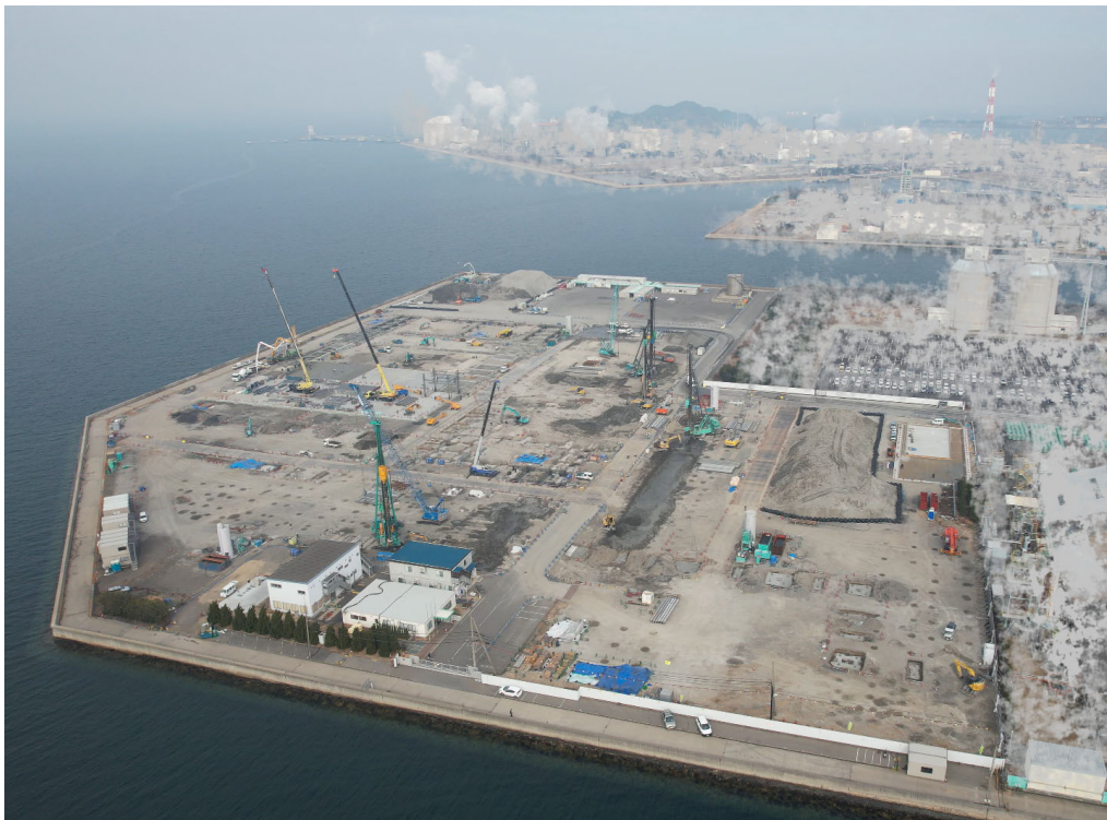
【New Plant of Battery Materials in Japan (Under Construction)(Jan. 2023)】
