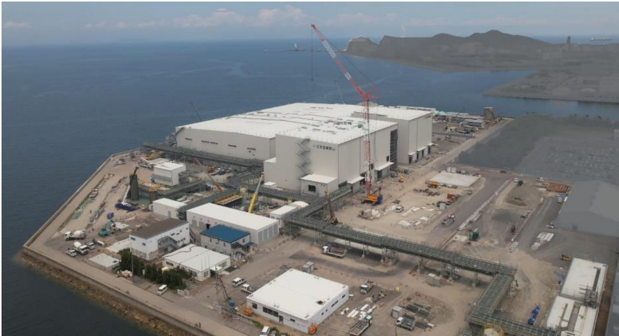
【New Plant of Battery Materials in Japan (Under Construction)(July 2023)】
