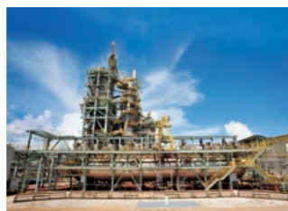
View of the Taganito HPAL Plant
