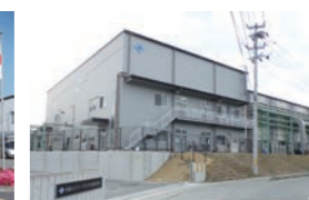
Sumiko Energy Materials Co., Ltd. Naraha Plant
