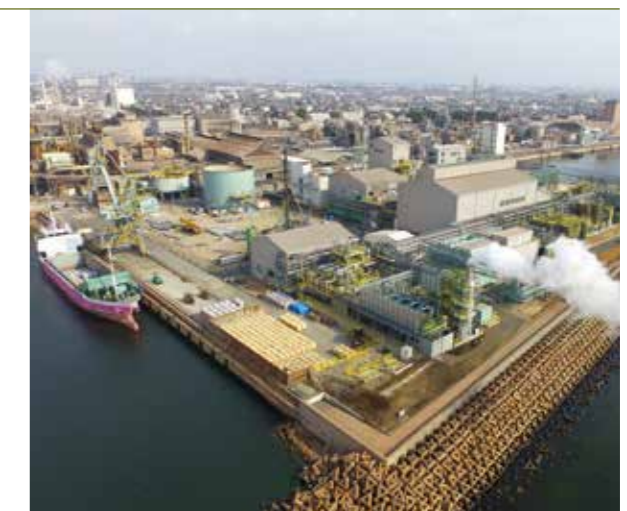
The Harima Refinery. A new battery materials precursor production plant is under construction.
