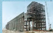
Toyo Smelter and Refinery under construction
