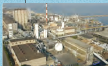
Toyo Smelter & Refinery
