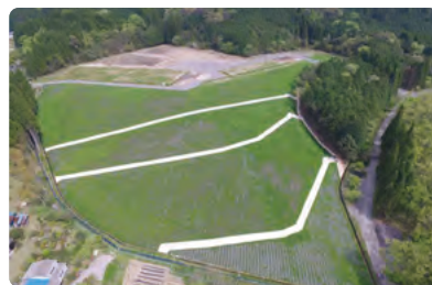
Greened state following the work
