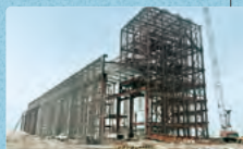
Toyo Smelter and Refinery under construction
