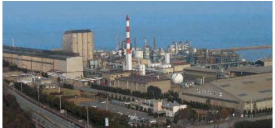
Toyo Smelter & Refinery
