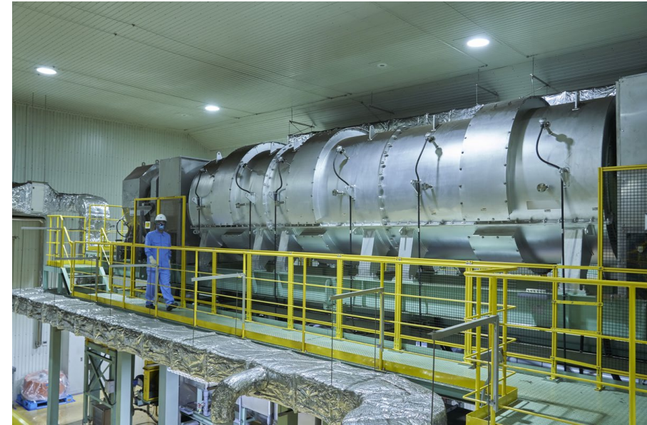
Isoura Plant (Ehime) for manufacturing battery cathode materials
